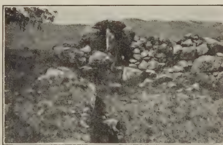
13. West wall of north tower (T1)
